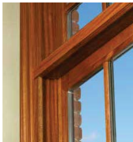
Concealed wood jamb liners provide a clean look
