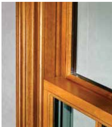
A wood wrapped jamb liner closure on the interior (shown) and an extruded aluminum jamb liner closure on the exterior hide the PVC jamb liners.
